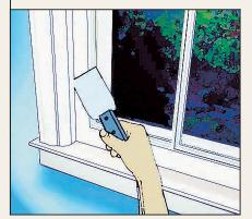
Outside, be sure to slide your putty knife between the bottom rail of the sash and window sill and pry gently. That's a common problem
